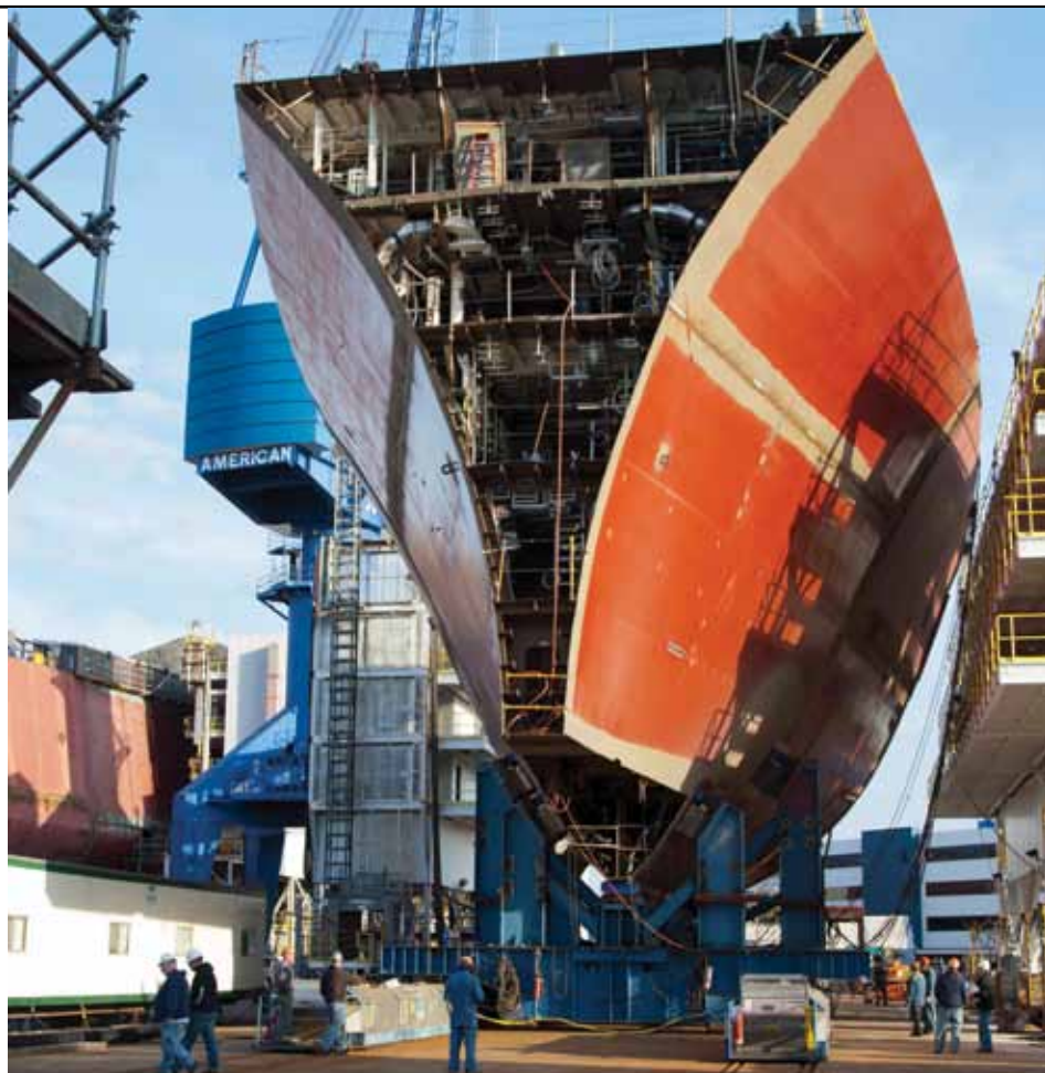
The DDG 115 Ultra Unit 1000 was transferred south onto Shipway 2 on September 20, 2014.
