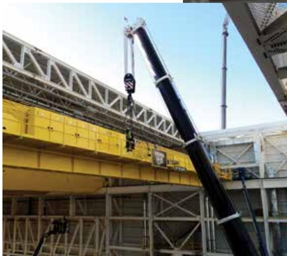
**9.** With the last girder of the West Crane landed, all four girders were in place.
