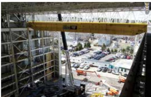
**8.** The East Crane ready to receive its two trolleys, each with a 100-ton and 25-ton hoist.
