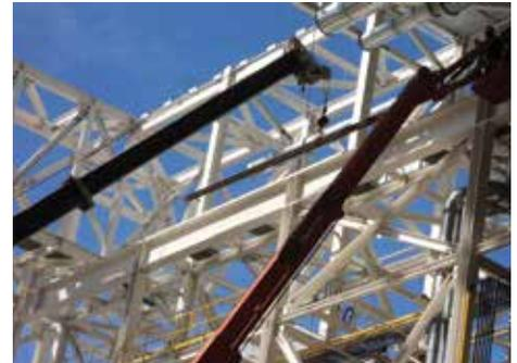
**3.** The crane runways were installed with part of the roof open to accommodate the 550-ton crane which would raise the girders 83 feet aloft. The installation was staged in West Bath.
